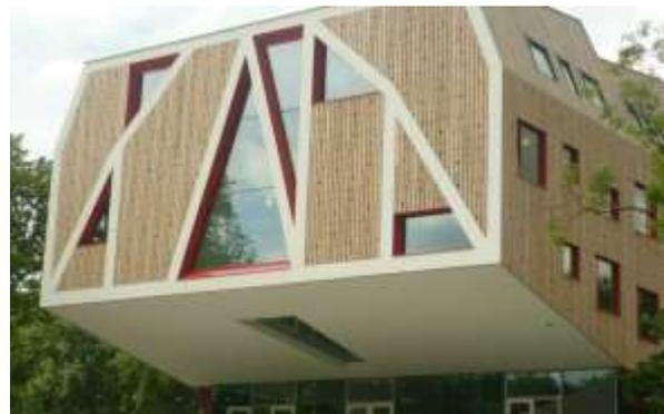
Fig. 4: The white parts are clad with Cempanel
