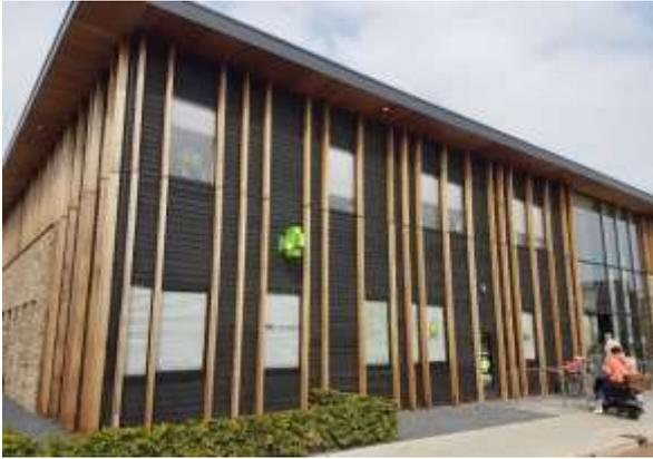
Fig. 5: The black wooden parts are coated with Xyhlo
