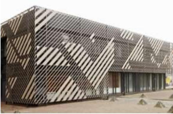
Fig. 1: Building with Resyta facade
